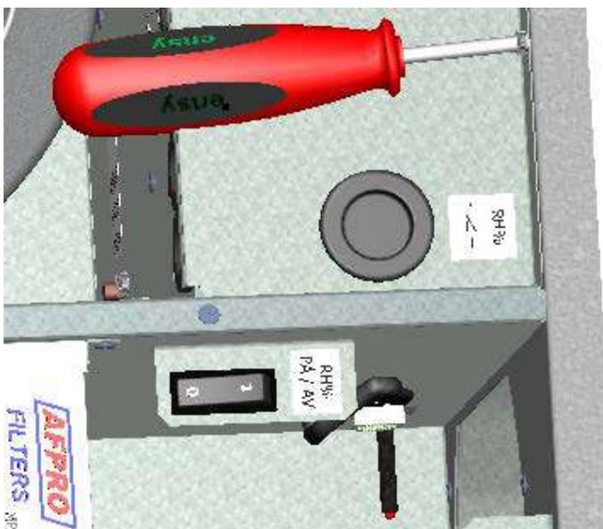
If it is necessary to adjust the sensitivity of the humidity sensor then you just can remove the black plug and you then can see the adjusting knob and the RH% scale.
