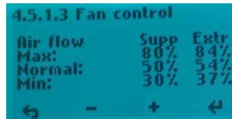
The installer can adjust these settings so that it is adequately balanced ventilation.
