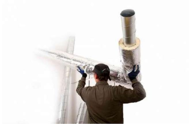
It can also be used insulation tubes (100 mm mineral wool) with plastic diffusion barrier pulled over the ducts. The same applies to insulation of pipings between the unit and diffusers, bringing the cooled air up to the rooms.
